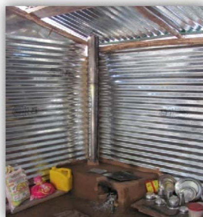
Smokeless chula installed in the shelter of Uttam Ram at Kapkot
