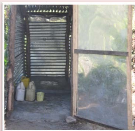
Toilet constructed for Dhanoli Devi
