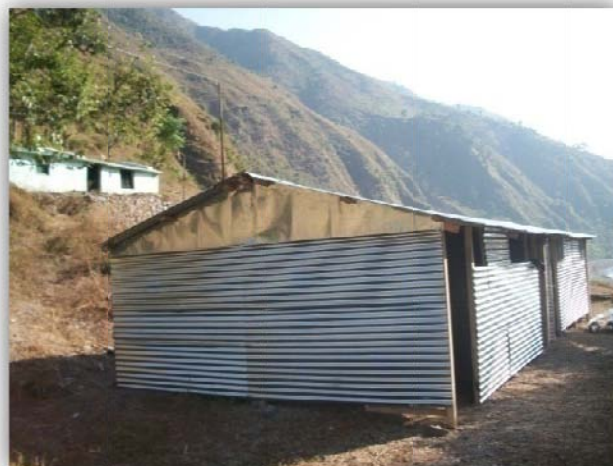
Construction of shelters in group of two families
